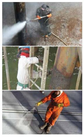
Surface preparation tolerance with excellent corrosion performance
